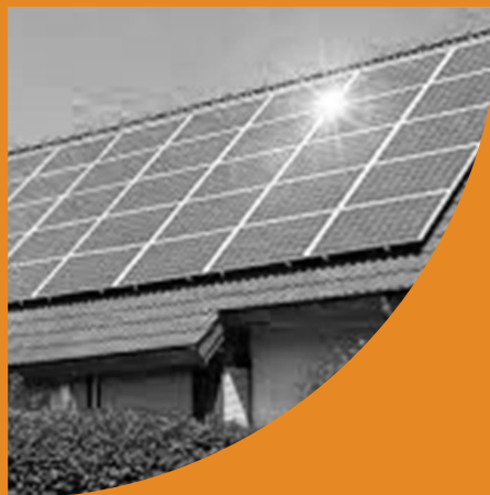
Solar Home System
